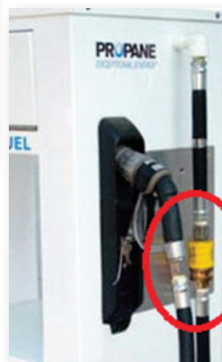
Poor installations, with restricted movement in direction of traffic
