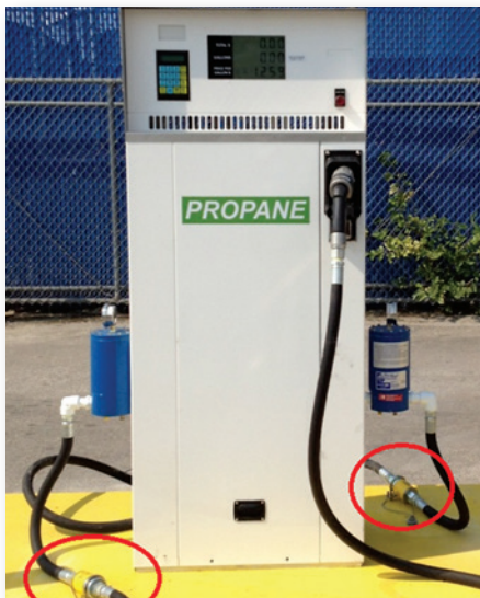
Good installation, with freedom of rotation
