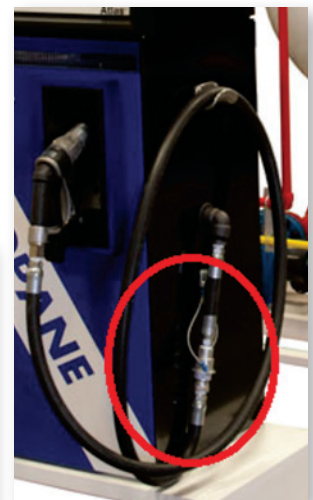
Poor installations, with restricted movement in direction of traffic
