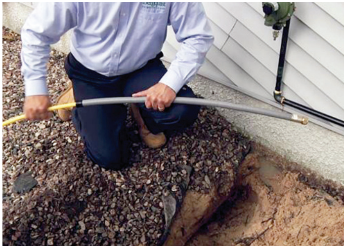
A technician installs a flex riser to protect the poly tubing above grade.
